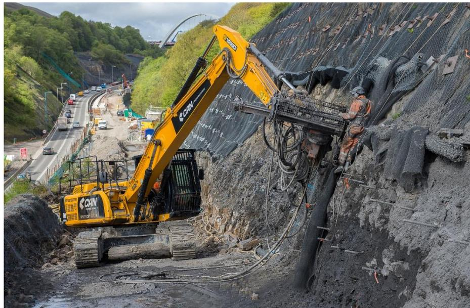
*Drilling work taking place with an excavator mounted drill rig*
